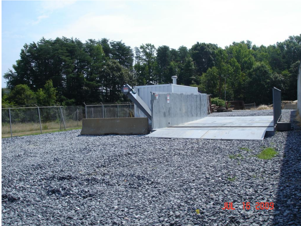
Marine Corps, (CIBRF) with conveyor (left side). Drive thru configuration Filtration equipment and pressure washer installed in all-weather enclosure Rack installed on slightly improved surface
